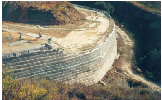
Mechanically stabilised earth (MSE) wall construction
