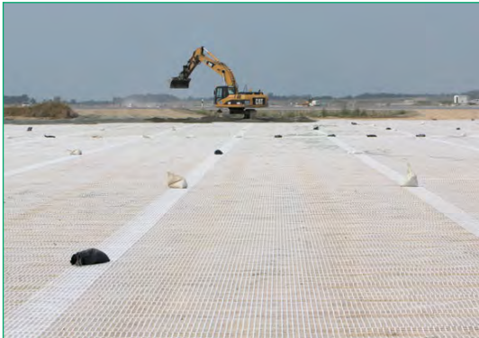
Fig. 7 Installed Secugrid® as a base course reinforcement
