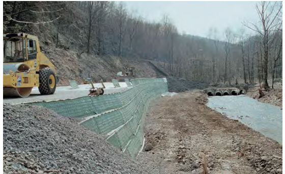
Railroad slope stabilisation
