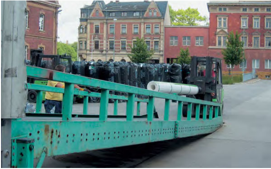
Loading of Secugrid®
