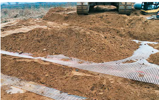
Two layers of Secugrid® as a road dam reinforcement
